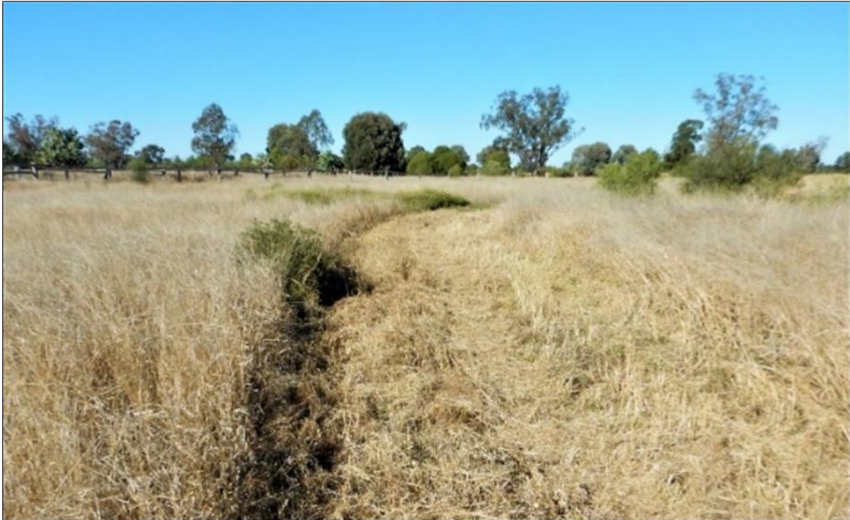
Figure 3-15: Prepared Seismic Line Following use of Bobcat Mounted Vegetation Mulcher in Tall / Dense Pasture Grass
