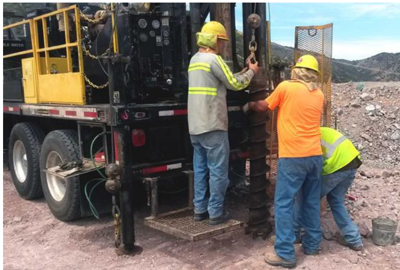
Figure 3-11: Truck Mounted Uphole Drilling Rig
