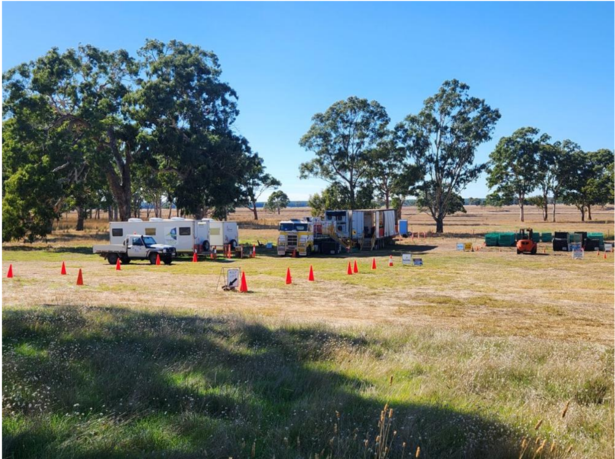
Figure 3-16: Seismic Survey Laydown Area (Source: Wayne M, 2026)
